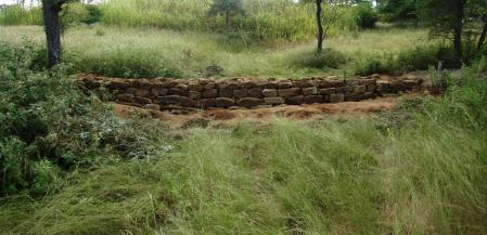
Check structures (made of stone, Do-Nou, brush-wood) for the purpose to control run off velocity so that not only soil conserved but also more rain water recharged as underground moisture)
