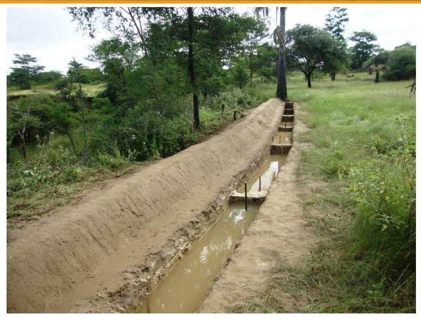
Small earth dam (embankment and spillway reinforced with Do-Nou) (to conserve soil + to capture more rain water so that stored as soil moisture)
